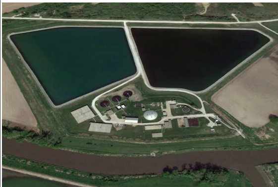
Aerial view of the DMU Wastewater Treatment Plant.
